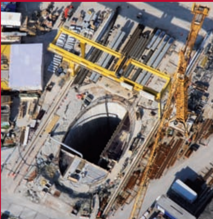
The oval access shaft, 35 m deep
