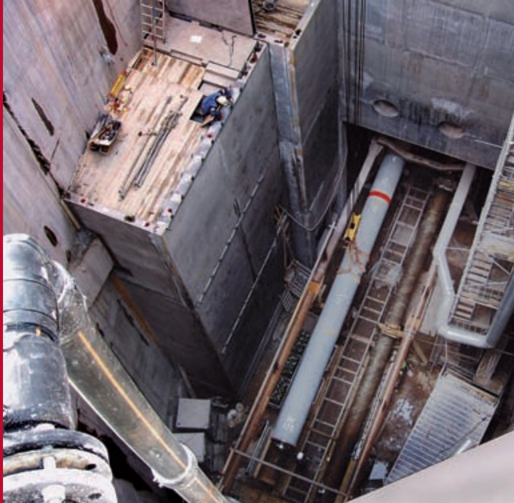
Looking down to one of the three tunnel shafts. The district heating pipes were lowered into them and then welded together.
