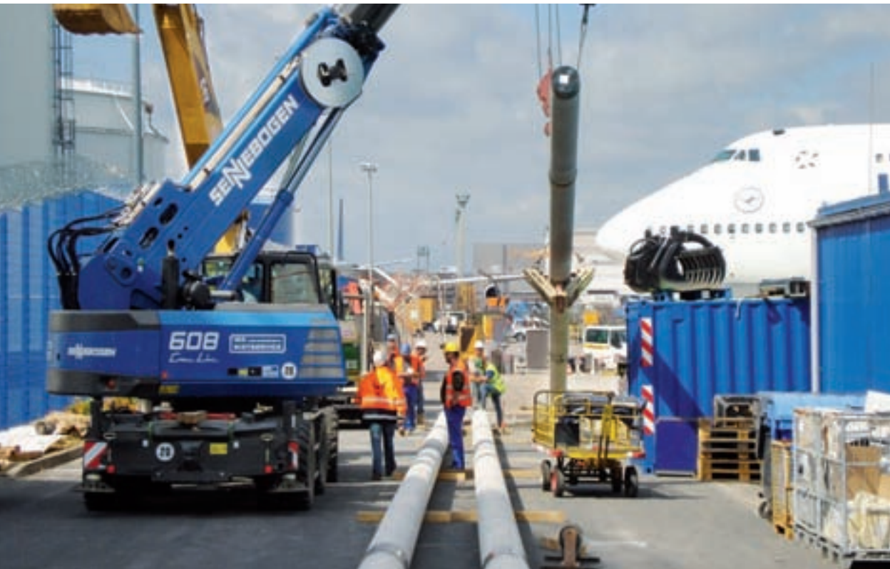
Pipe-laying operations by the Nacap company at Frankfurt Airport
