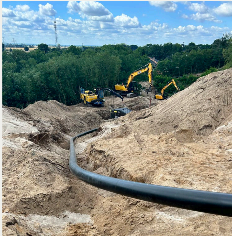
Pipe-laying took place in some cases on challenging terrain.
