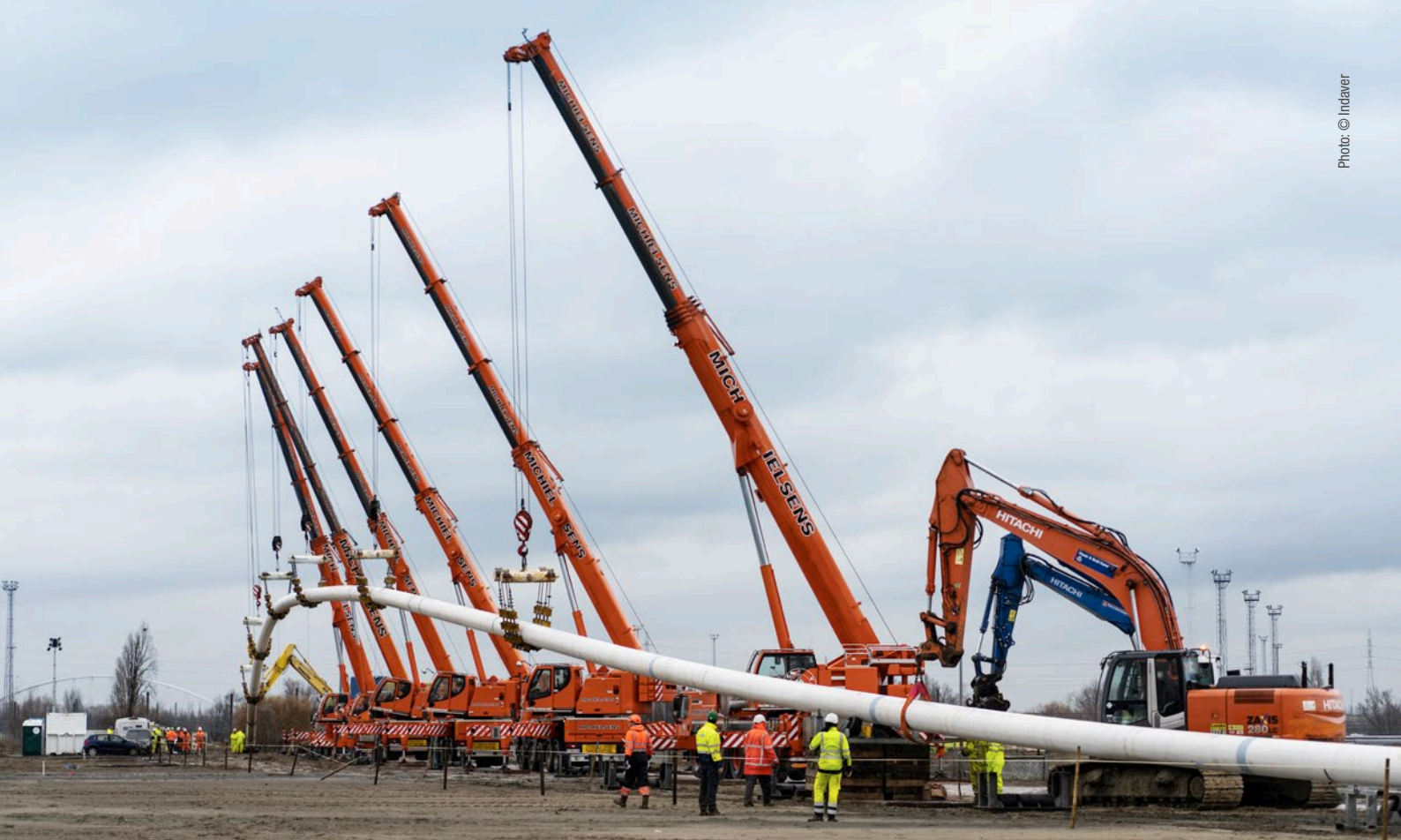
Pipe laying for the “Warmtenetwerk Antwerpen Noord”
