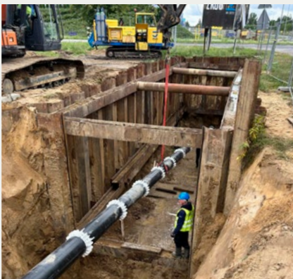
Preparations for a pipeline passing under a road.
