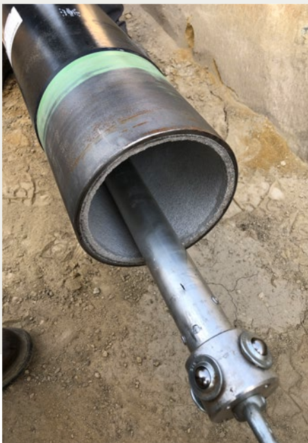
Pigging device lance for pipe joints.
