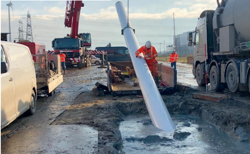
The PP-coated pipes are guided into the prepared trench.
