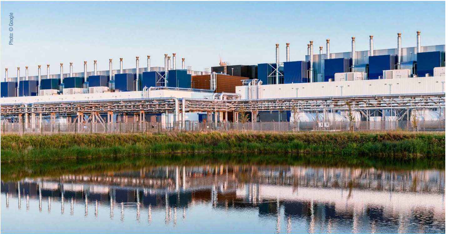
The Google data center in Eemshaven resembles an industrial complex from the outside.
