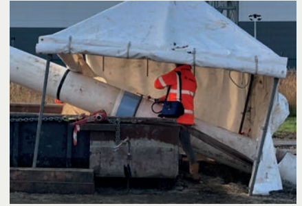
Testing of the field coating and welded joint.
