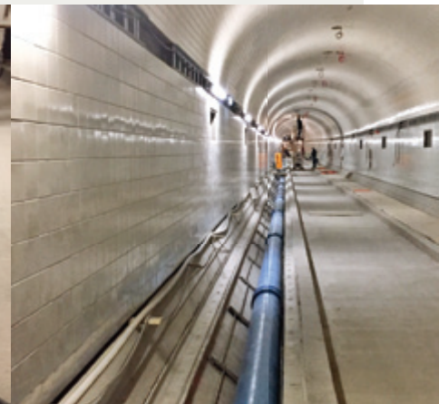
The 426.5 m long pipeline was installed completely without welding.
