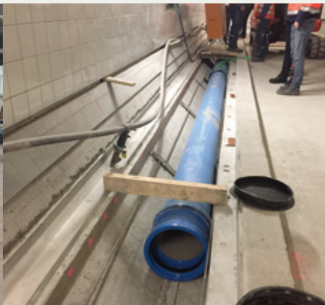
The HFI-welded steel pipes (DN 300) fitted precisely into the prepared ducts.
